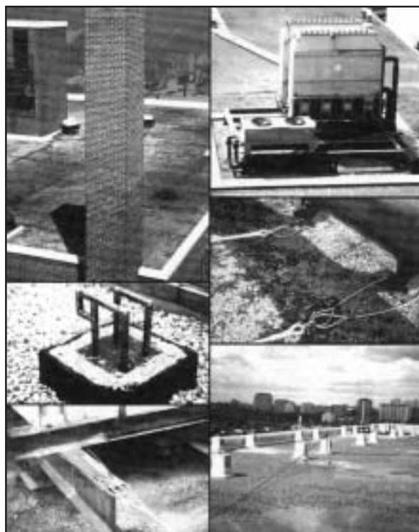
Examples of adequate anchorage
