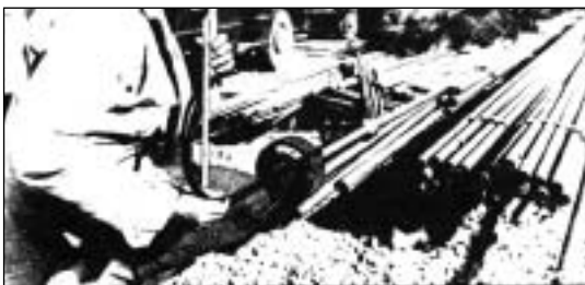
Figure 1.17: Bundles of bar tendons stored on dunnage
