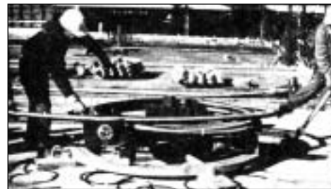
Figure 1.21 Cutting bands progressively, and crew of rodworkers using the uncoiling turntable
