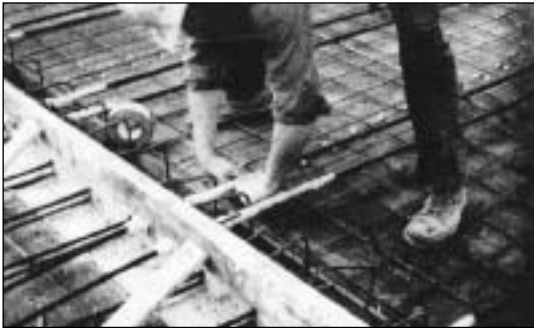
Figure 1.19 Taping around casting, connector, and strand
