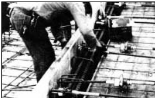
Rodworker attaching anchorage assembly to forms
