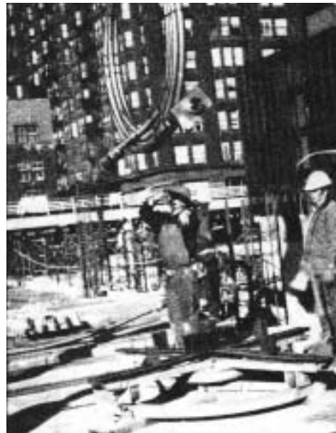
Figure 1.20 Rigging tendon with nylon slings being lowered on field tendon uncoiler
